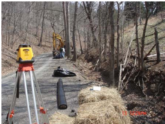
Site during construction.
